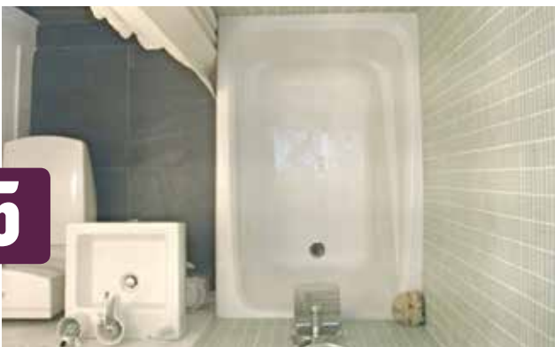
5 Small bathrooms and ensuites with insufficient circulation space
