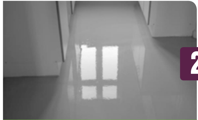
2 High gloss potentially slippery floor tiles
