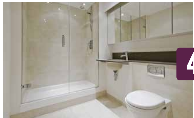
4 Large steps at the shower entry point
